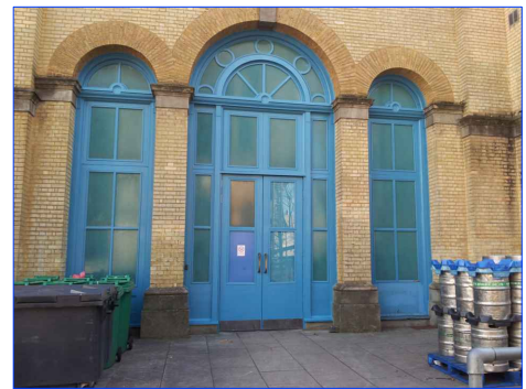
Fig. I. Restored windows to Palm Court, Alexandra Palace
